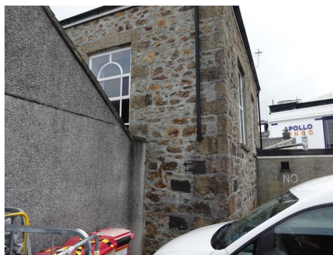
18. Missing downpipe sections southwest corner.
