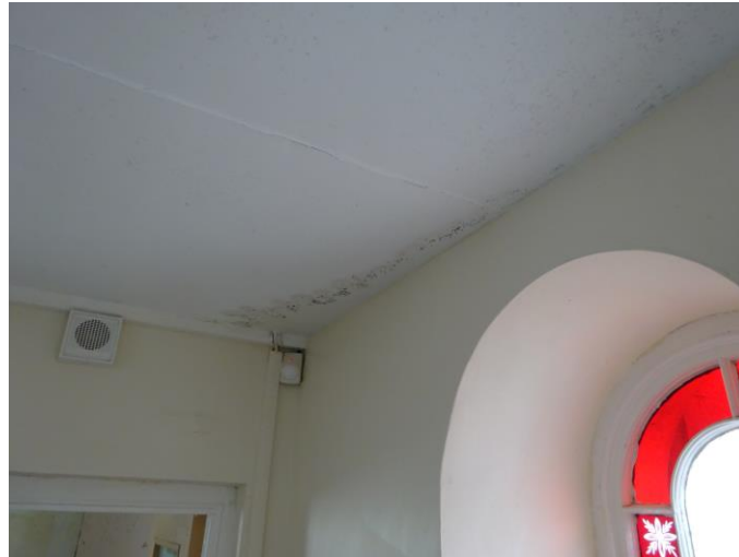
42. Damp stain to east corridor north side.
