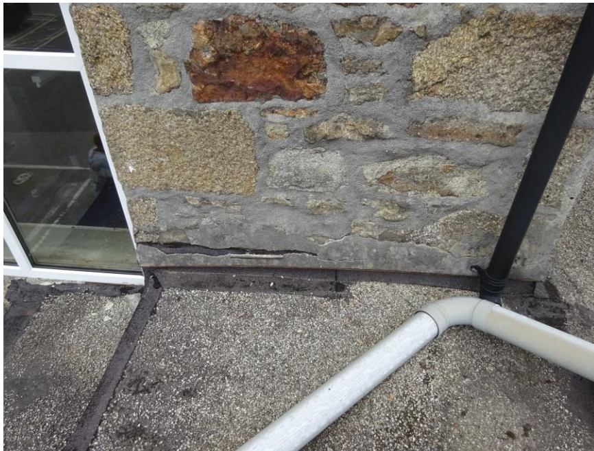
28. Defective weathering from flat roof to Wall 8.
