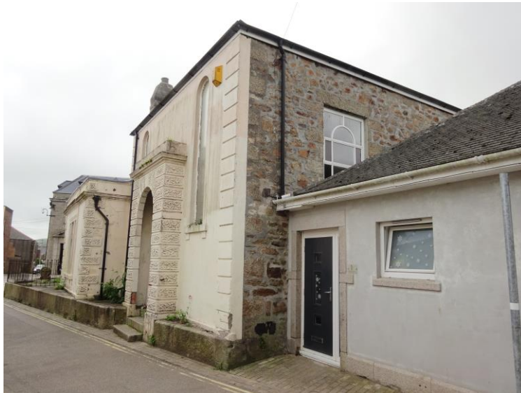
2. View along north elevation with Wall 1 and R1 fascia.
