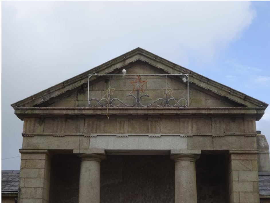
27. View of pediment – note Christmas lights.
