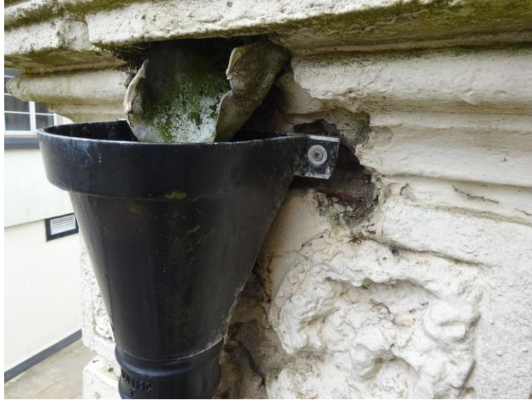
19. Hopper to west end of R5
