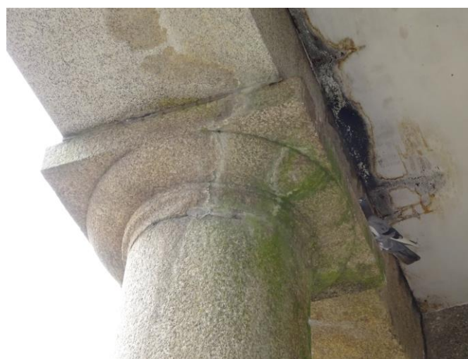
26. South column and boarding.
