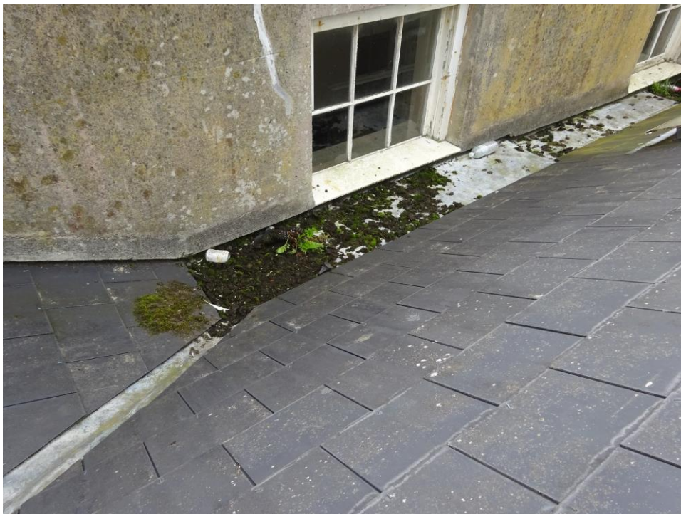
16. Lead valley to R5 south side.
