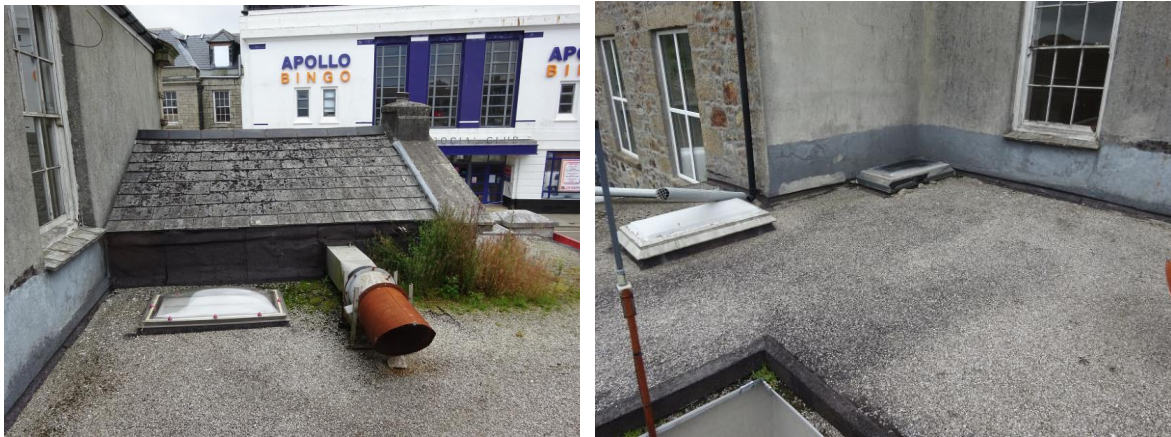
12. Dome skylights to flat roof
