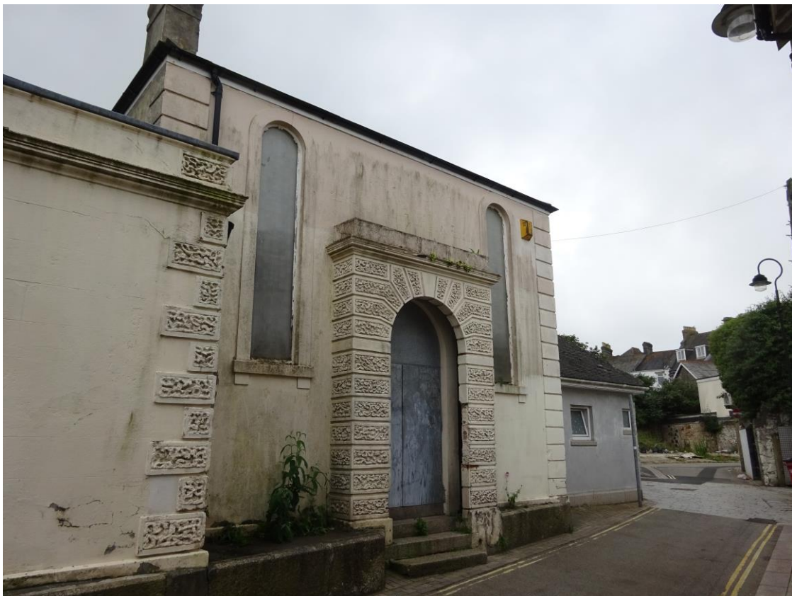
22. North wall of western hall.
