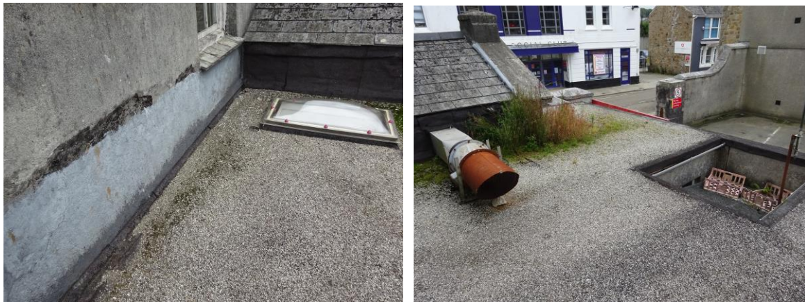
11. Flat roof to south side
