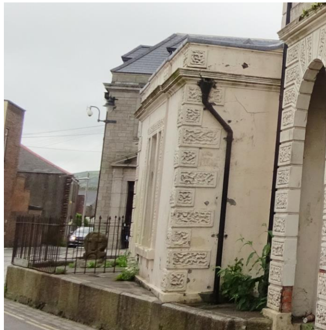
20. DP below hopper as per picture 19.
