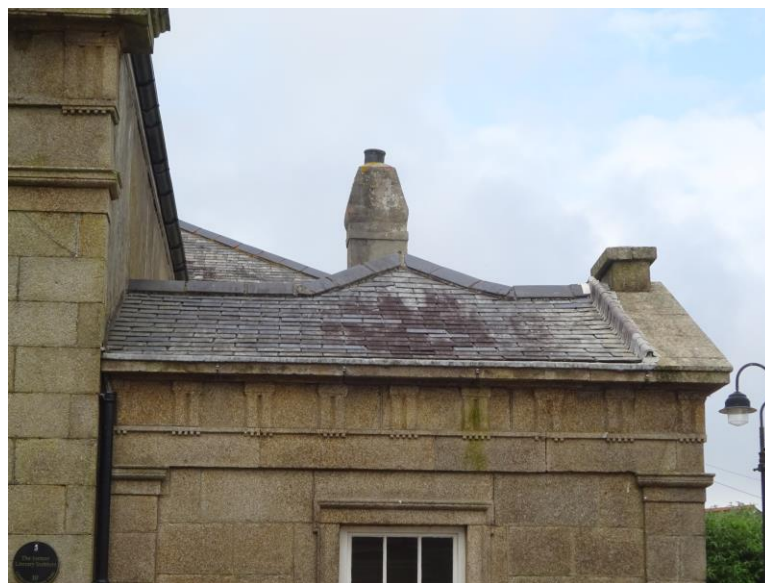
5. R3 from east
