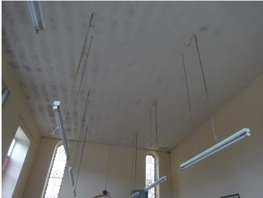
40. Ceiling to western hall.
