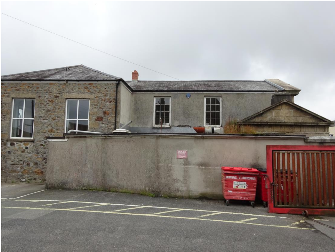
29. View of south elevation wall.
