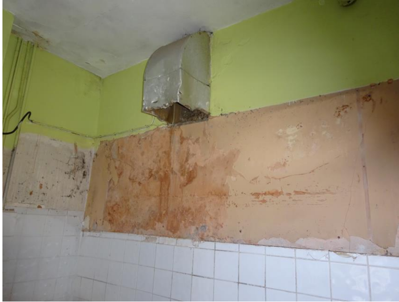
41. West wall of south kitchen.
