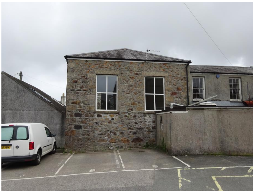
30. South side of western hall showing windows W4 and W5.
