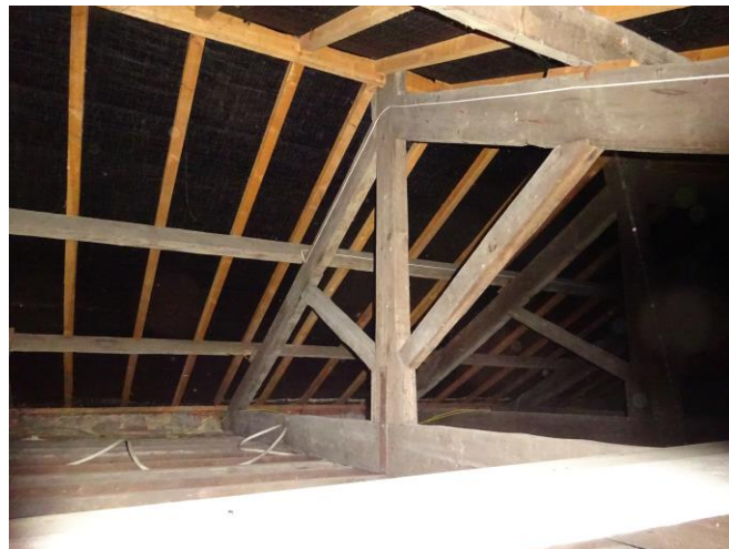
36. R2 roof void.
